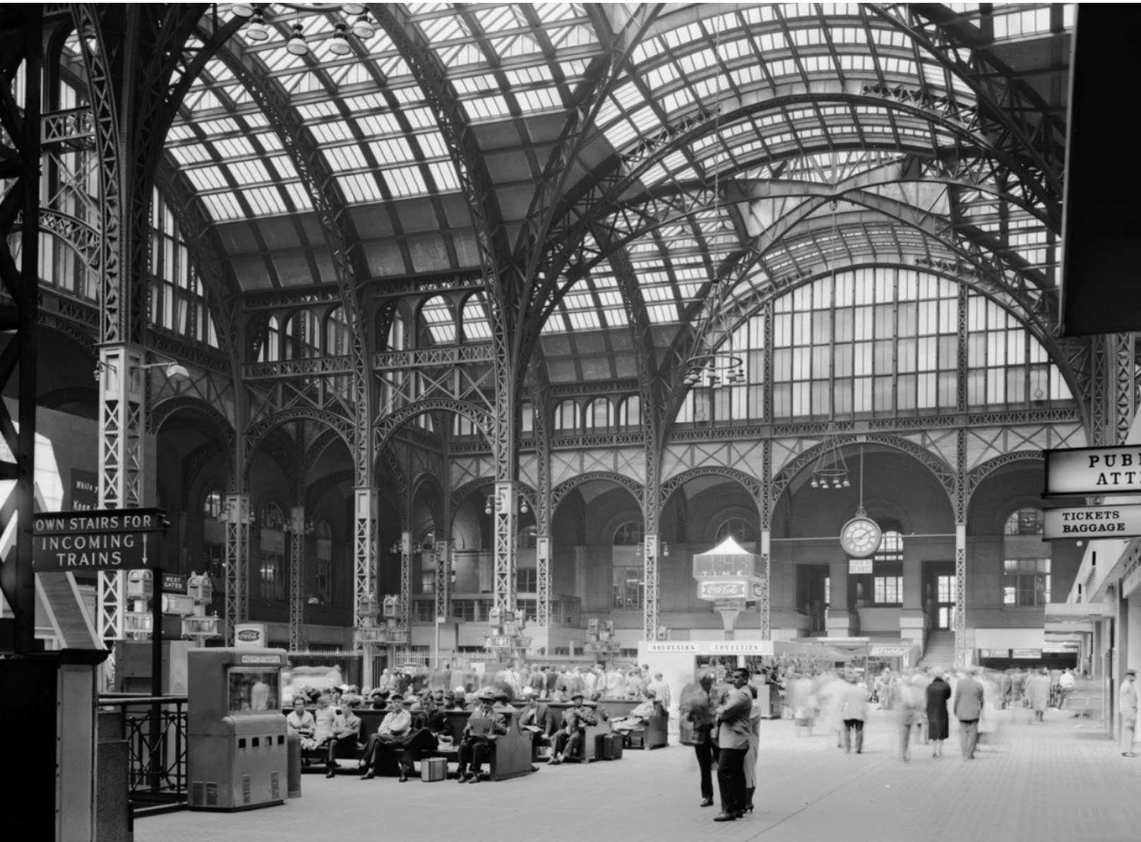
New York-Pennsylvania Station Architects: McKim, Mead, and White Photo (1935) by Berenice Abbott ©New York Public Library
